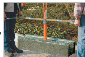
Posa cordoli e canali Kerb and curbstone laying
